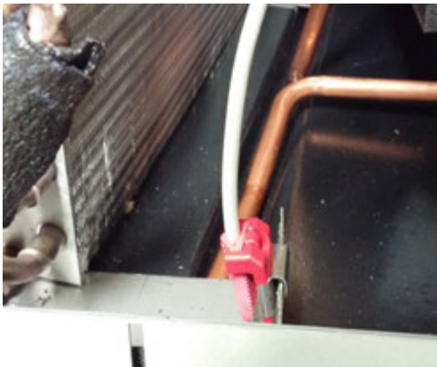
FIGURE 35 Outdoor Condensate Sensor
