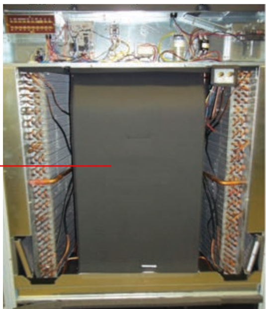
FIGURE 4 Removal of Air Duct
