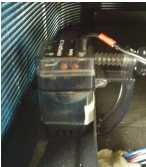
FIGURE 19 Outdoor Condensate Sensor
