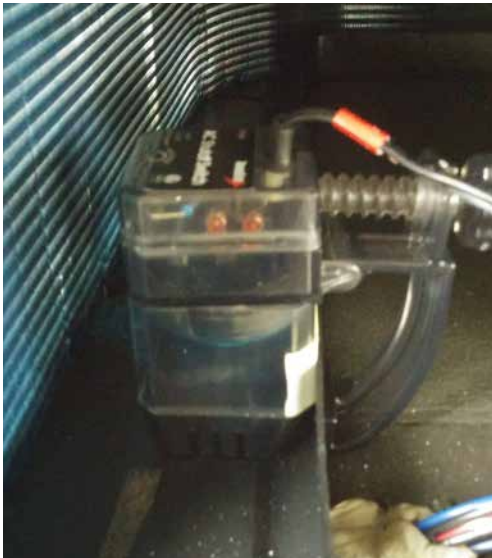
FIGURE 35 Outdoor Condensate Sensor
