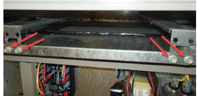
FIGURE 6 Remove Four Screws
