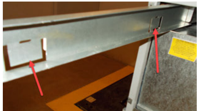
FIGURE 37 Bend Filter Tabs Down
