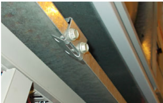
FIGURE 40 Re-Install Screws and Bend Tabs Up
