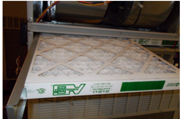
FIGURE 42 Install Left 2" Filter
