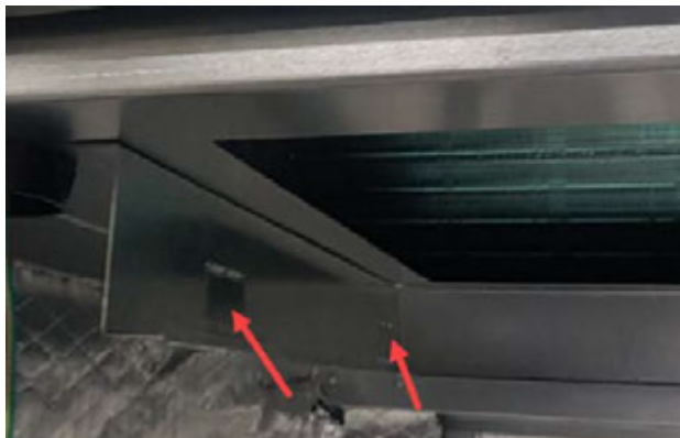
FIGURE 10 Bend Filter Tabs Down
