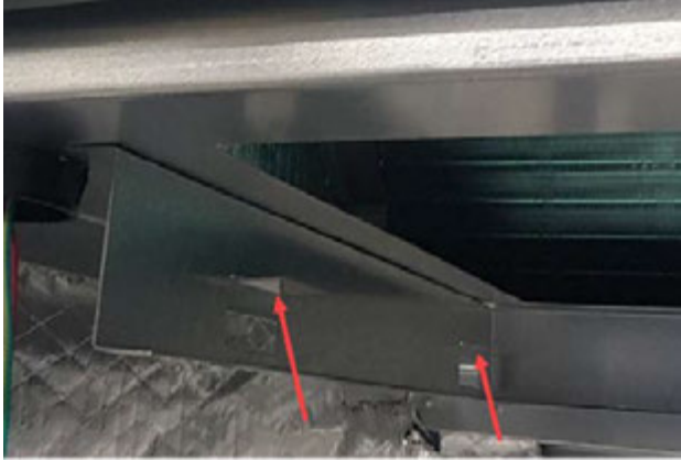
FIGURE 10 Bend Filter Tabs Down
