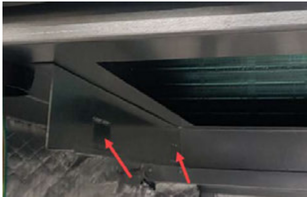
FIGURE 10 Bend Filter Tabs Down
