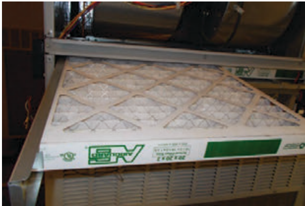
FIGURE 10 Install Left 2" Filter
