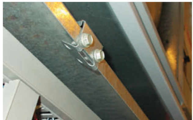
FIGURE 8 Re-Install Screws and Bend Tabs Up
