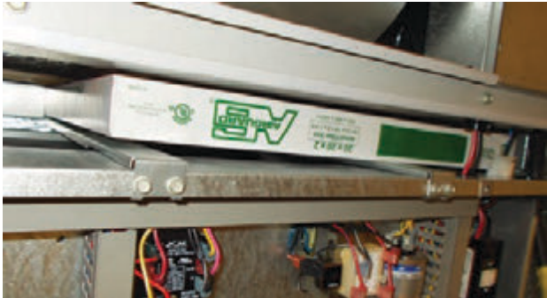
FIGURE 10 Install Left 2" Filter
