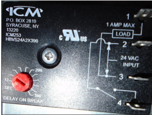
FIGURE 4 Exhaust Fan Off Delay Timer
