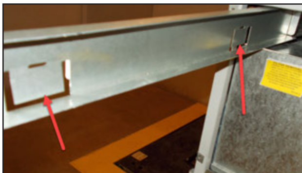
FIGURE 62 Bend Filter Tabs Down
