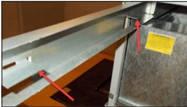
FIGURE 61 Filter Tabs in Up Position
