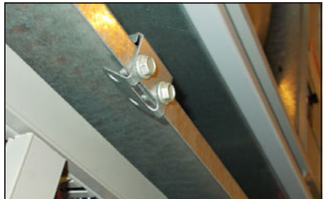
FIGURE 65 Re-Install Screws and Bend Tabs Up
