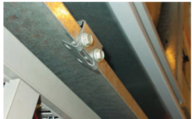
FIGURE 8 Re-Install Screws and Bend Tabs Up
