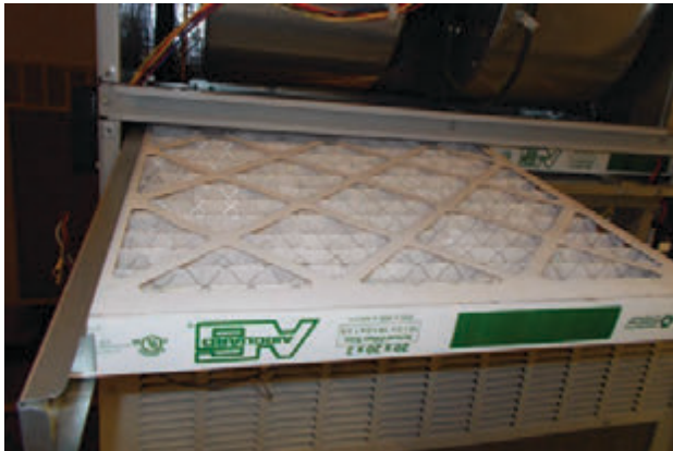
FIGURE 10 Install Left 2" Filter
