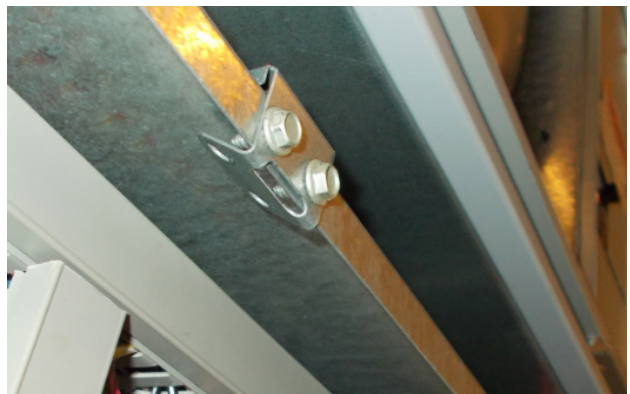
FIGURE 8 Re-Install Screws and Bend Tabs Up
