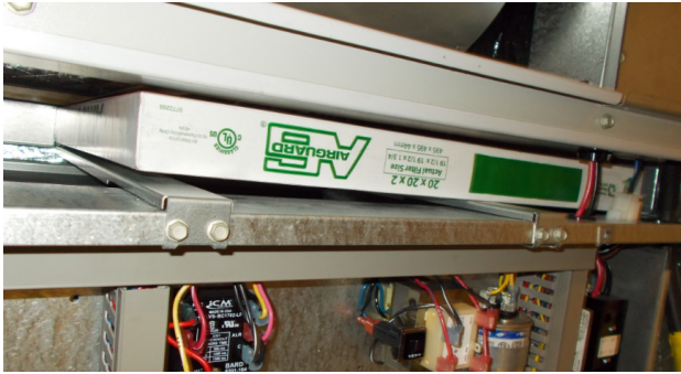
FIGURE 10 Install Left 2" Filter
