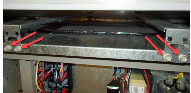
FIGURE 6 Remove Four Screws
