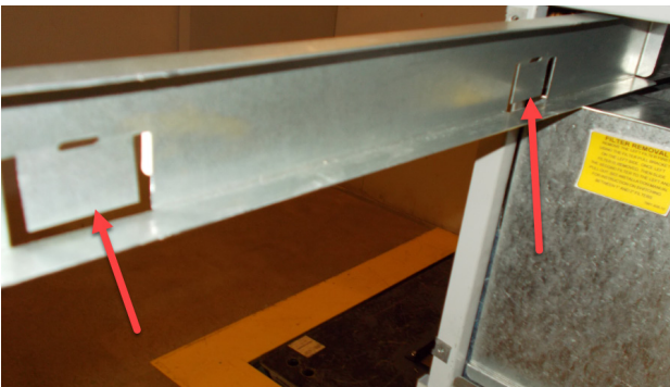
FIGURE 5 Bend Filter Tabs Down
