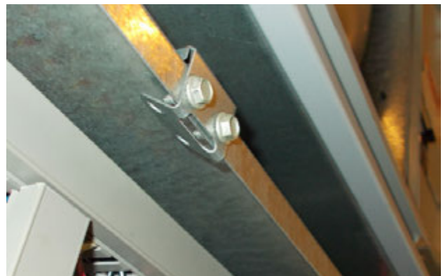
FIGURE 8 Re-Install Screws and Bend Tabs Up
