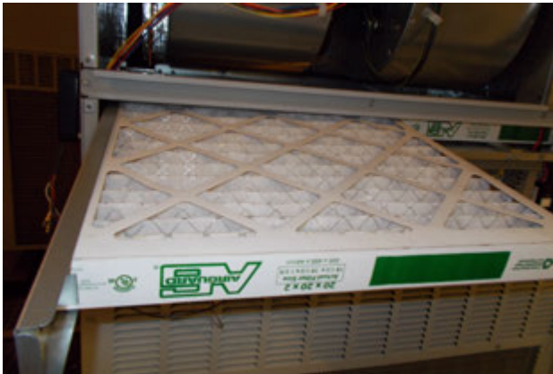
FIGURE 10 Install Left 2" Filter
