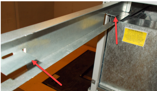
FIGURE 4 Filter Tabs in Up Position
