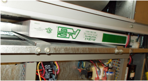
FIGURE 10 Install Left 2" Filter
