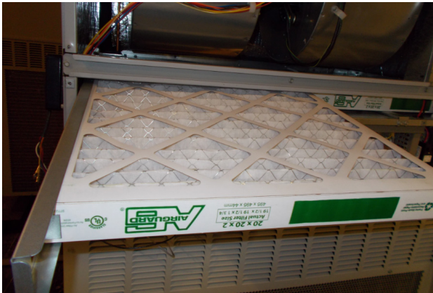
FIGURE 10 Install Left 2" Filter
