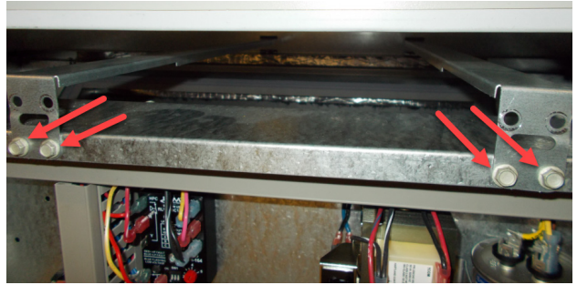
FIGURE 6 Remove Four Screws
