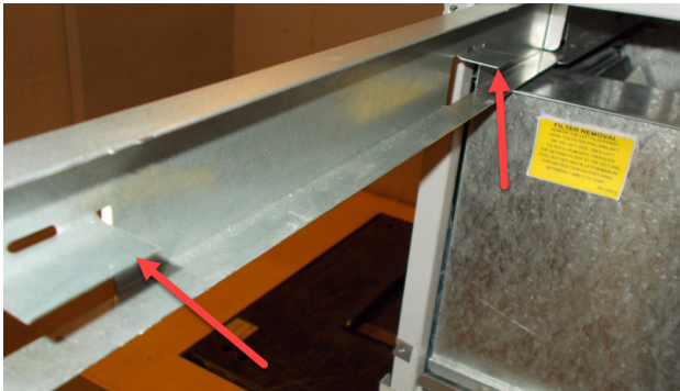
FIGURE 4 Filter Tabs in Up Position
