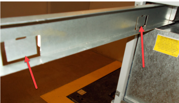
FIGURE 5 Bend Filter Tabs Down
