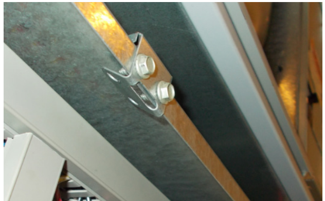
FIGURE 8 Re-Install Screws and Bend Tabs Up
