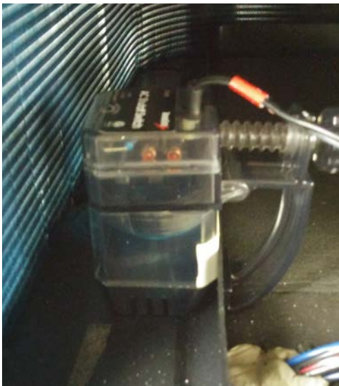
FIGURE 19 Outdoor Condensate Sensor
