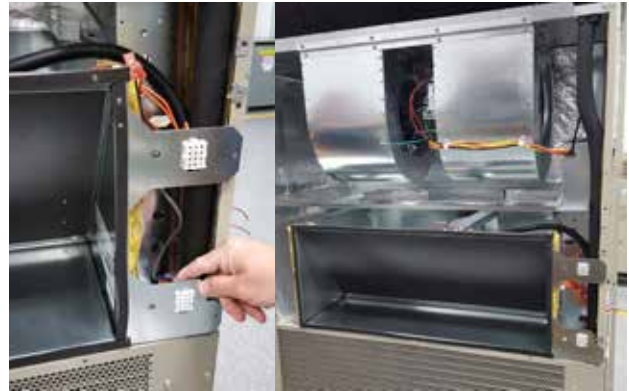
FIGURE 14 Orange Wires Routed Along Refrigerant Lines
