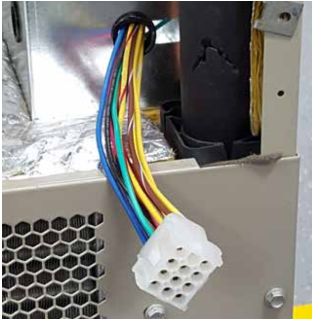
FIGURE 12 Low Voltage Wire Harness Pulled Through Grommet
