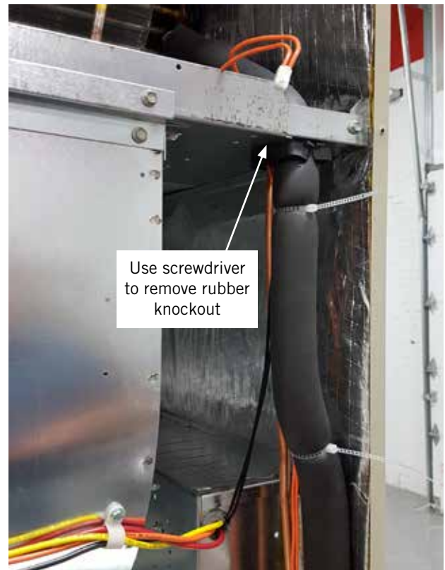
FIGURE 14 Orange Wires Routed Along Refrigerant Lines
