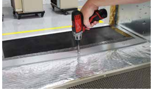
FIGURE 4 New Condenser Exhaust Plate with Screen Installation
