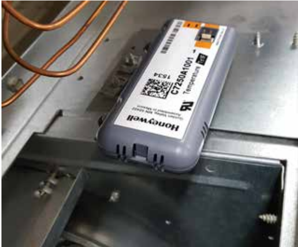
FIGURE 16 Mixed Air Temperature Sensor Location
