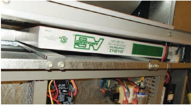
FIGURE 10 Install Left 2" Filter
