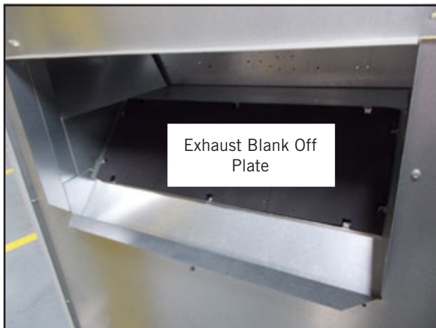
FIGURE 5 Remove Exhaust Blank Off Plate
