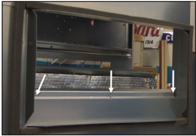
FIGURE 28 Install Rear ERV Mounting Rail
