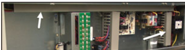
FIGURE 23 Remove Two Wire Channel Covers
