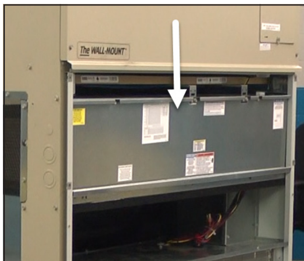
FIGURE 3 Remove Low Voltage Control Panel
