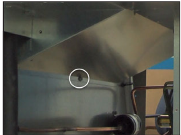
FIGURE 7 Remove Screw from Condenser Partition Insert
