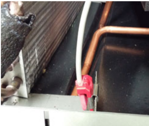
FIGURE 35 Outdoor Condensate Sensor
