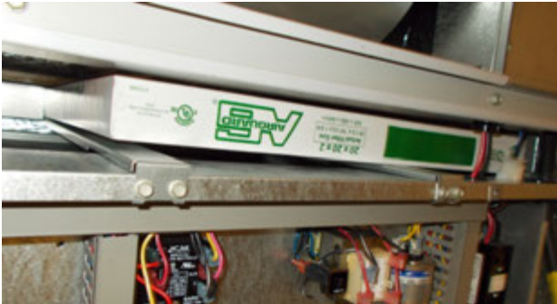
FIGURE 10 Install Left 2" Filter
