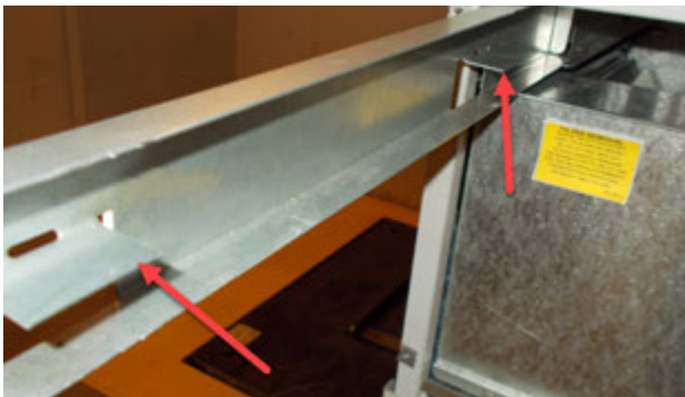
FIGURE 4 Filter Tabs in Up Position
