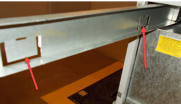
FIGURE 5 Bend Filter Tabs Down
