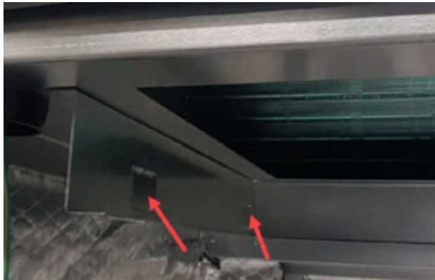
FIGURE 10 Bend Filter Tabs Down
