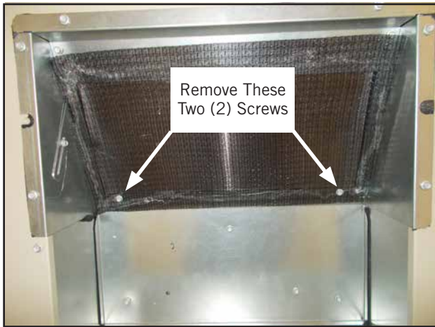
FIGURE 8 Remove Blade Screws
