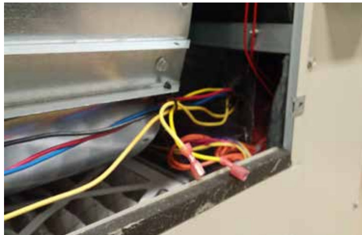
FIGURE 4 Freeze Stat Wire Routing
