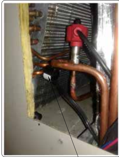
FIGURE 3 Freeze Stat Location and Wire Routing
