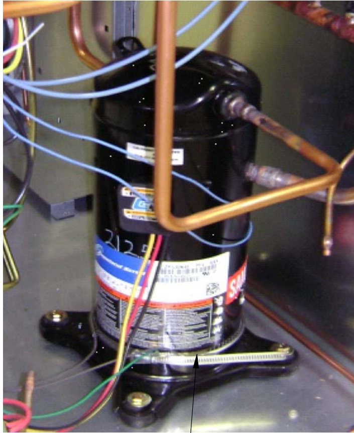
FIGURE 1 Attaching Crankcase Heater to Compressor
