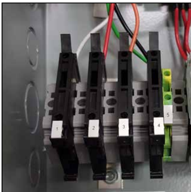
FIGURE 2 LC6000 Fused Power Supply Terminals
