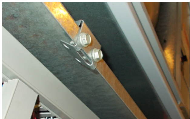
FIGURE 8 Re-Install Screws and Bend Tabs Up
