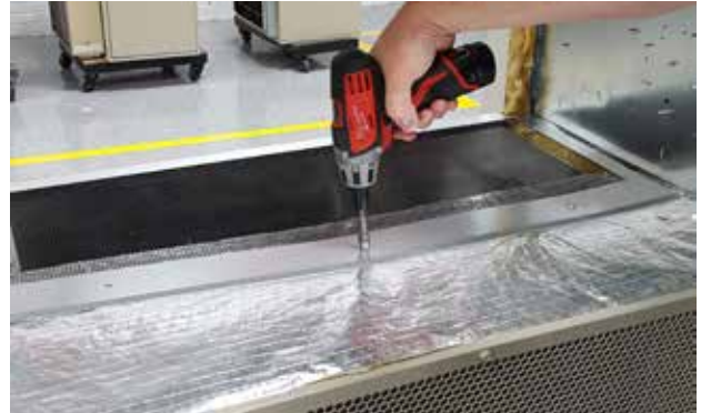
FIGURE 4 New Condensor Exhaust Plate with Screen Installation
