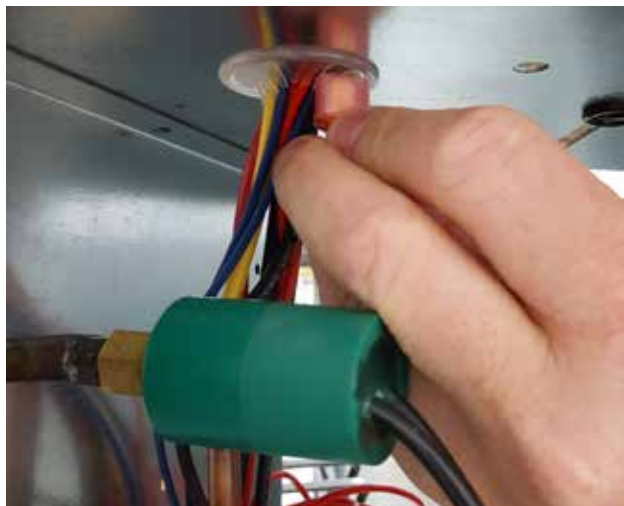
FIGURE 11 Wire Harness Through Grommet
