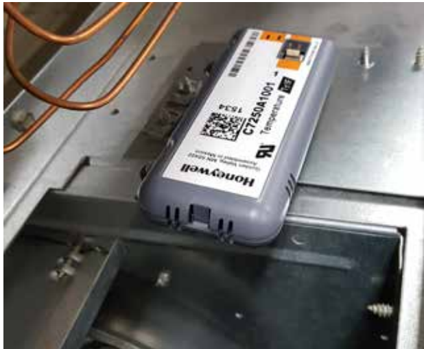
FIGURE 16 Mixed Air Temperature Sensor Location
