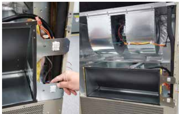
FIGURE 14 Orange Wires Routed Along Refrigerant Lines
