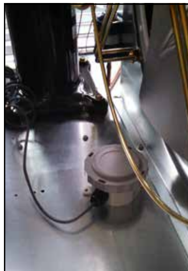
FIGURE 3 Outdoor Sensor Installation
