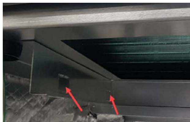
FIGURE 10 Bend Filter Tabs Down
