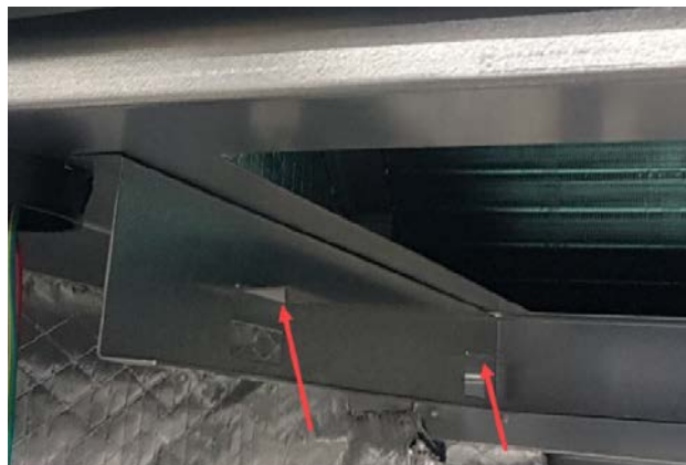
FIGURE 10 Bend Filter Tabs Down
